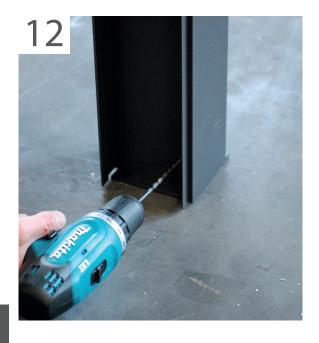
Once the gutter has been aligned horizontally, drill holes and screw in the posts. Now you can proceed with the roof supports.
