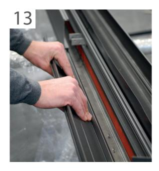
Click the gutter risers out of the gutter by pulling them toward you. Mount the bracket 55 mm from the side of the gutter. Do this at both ends of the gutter. Drill a 75 mm hole for the drain if necessary.
