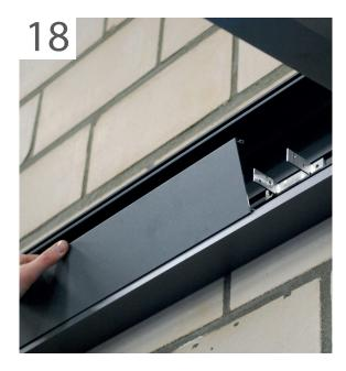
Once the side supports are installed, position the gutter riser directly against the side supports.
