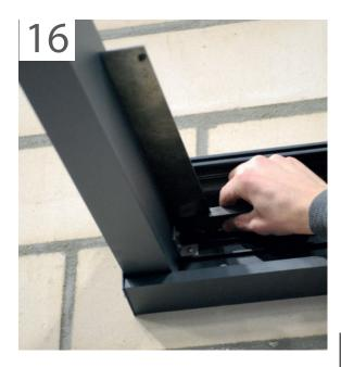
Make sure the roof is aligned squarely so that the beams are at right angles. If necessary, use a protractor or other method to determine squareness.
