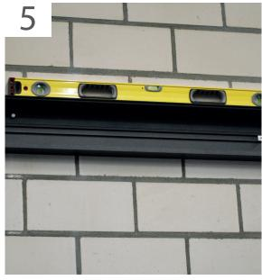
Ensure that the wall profile is positioned horizontally. Seal the top of the wall profile.
