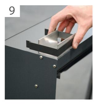
Screw the post brackets to the bottom of the gutter at the desired location. A strip can be sawn off the post as a drilling jig to determine the correct position of the bracket. Do not drill into the gutter box.
