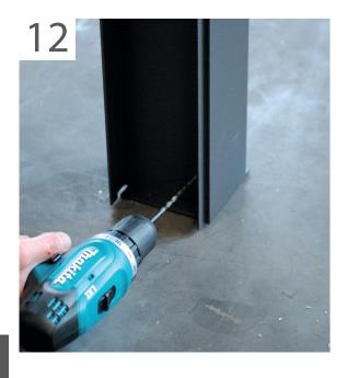
Once the gutter has been aligned horizontally, drill holes and screw in the posts. Now you can proceed with the roof supports.
