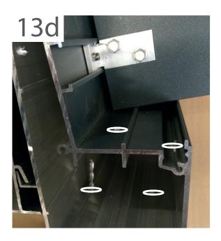
Drill drainage holes into the rear section of the gutter for possible condensation. The drainage holes must be placed at four locations at the height of the post.
