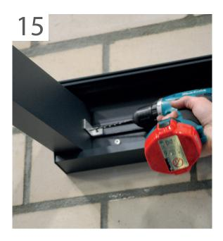
The side supports are screwed to the (half) brackets. Two screws are used per side to mount the intermediate supports in the brackets.
