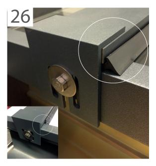
Position the buffer block on the plastic support and screw it in place. For a glass roof, leave the rubber protruding slightly; for a polycarbonate roof, leave it protruding slightly. Seal the side support.
