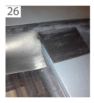
Now pull the wall rubber over the first pane and cut it at the height of the cover strips. Continue this process for the entire roof from left to right or vice versa. Cut the rubber in the gutter in the same way.
