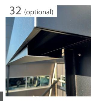
If INVIGO PRO is NOT installed, cover the opening in the gutter with a cover strip. Align it so that both sides fall behind the post sides and click it into the opening.
