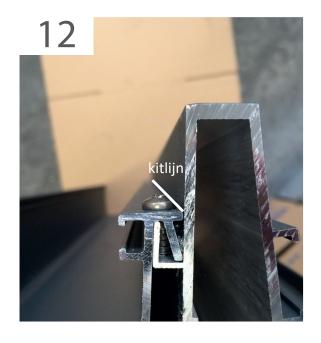
Seal the edge between the gutter box and the rear part of the gutter. Do this at the specified location.
