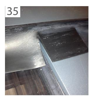
Now pull the wall rubber over the first pane and cut it at the height of the cover strips. Continue this process for the entire roof from left to right or vice versa. Cut the rubber in the gutter in the same way at the height of
