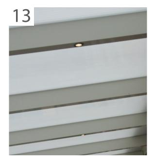
The holes for the Pallazzo LED spotlights are drilled with a diameter of 29 mm. Please refer to the wiring diagrams for wiring connections.
