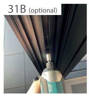
Place the guide profile in the corresponding opening, ensuring that both sides fit behind the post sides. Drill through the prepared holes in the first gutter wall and then screw the parts together.
